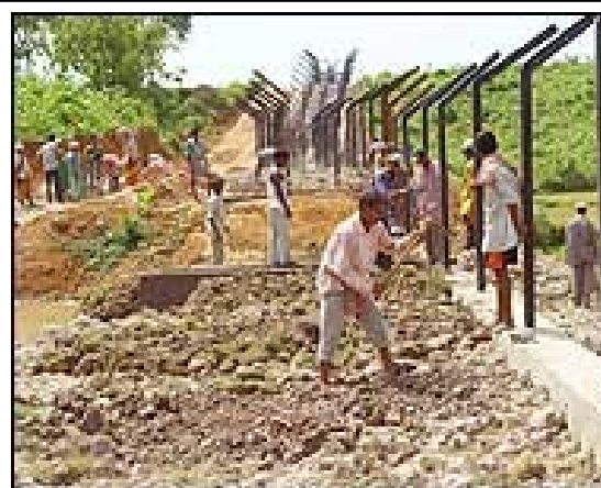
Figure 7.2 A view of the erection of fences across the Bangladesh border
